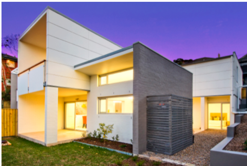
Architect house with cross-ventilation louvers to take advantage of ocean breezes Manly Beach, Sydney, Australia
