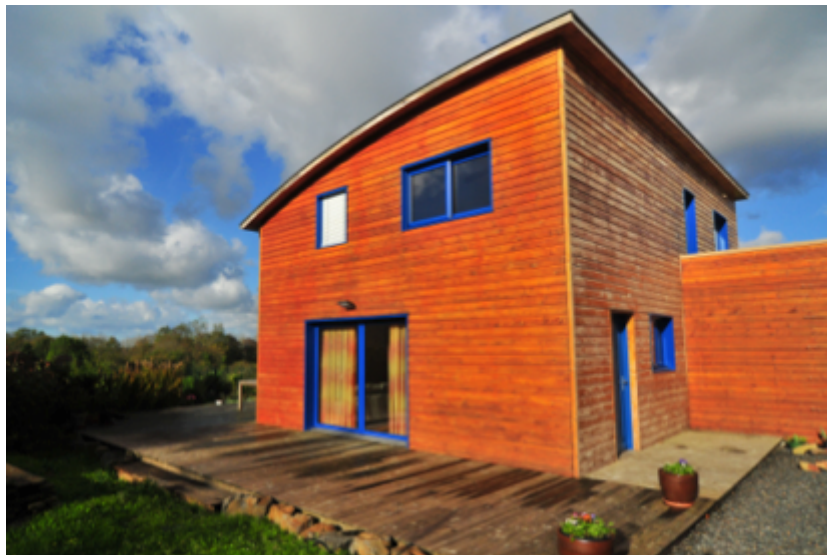
Brand new home with a green roof, entirely built with natural materials, just minutes from the D-Day beaches Bayeux, Normandy, France
